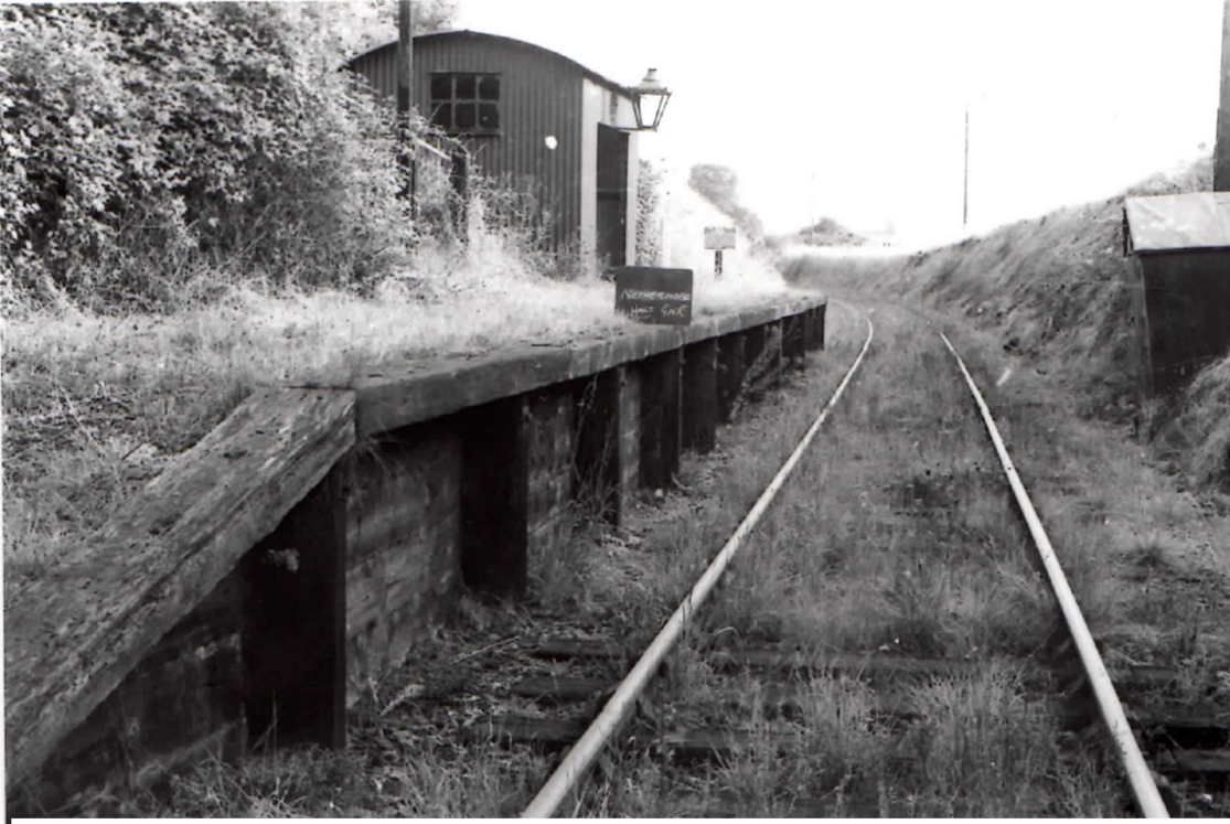
Netherhope Halt from the tunnel end. The bright steel of the rail surface indicates that Tintern quarry was still open. Apart from grass growing through the platform surface the halt looks to be in good condition. This dates the photograph as probably being in the early 1960s ( Lens of Sutton )
