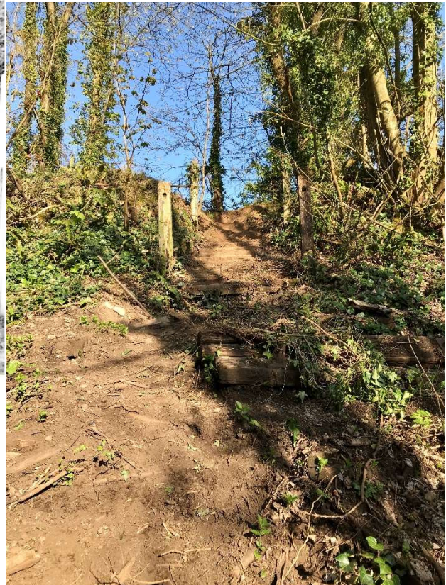
All that is left of Netherhope Halt April 2021: Some steps up the bank on the far side of the shelter and four posts that supported the hand- rails. (Martin Scott)
