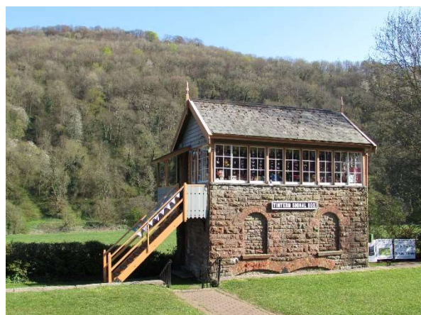
Signal box after restoration ( Michaelday_bath CC BY-NC 2.0 )
