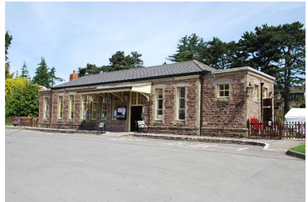
Forecourt rebuilt at Winchcombe ( Hugh Llewelyn CC BA-SA 2.0 )
