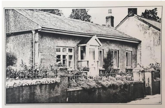
The Reading Room at Woodcroft, believed to be the former Baptist Meeting Room and Coffee Room run by the Morgan ladies ( Geoff Mead's papers courtesy of Tidenham History Group )
