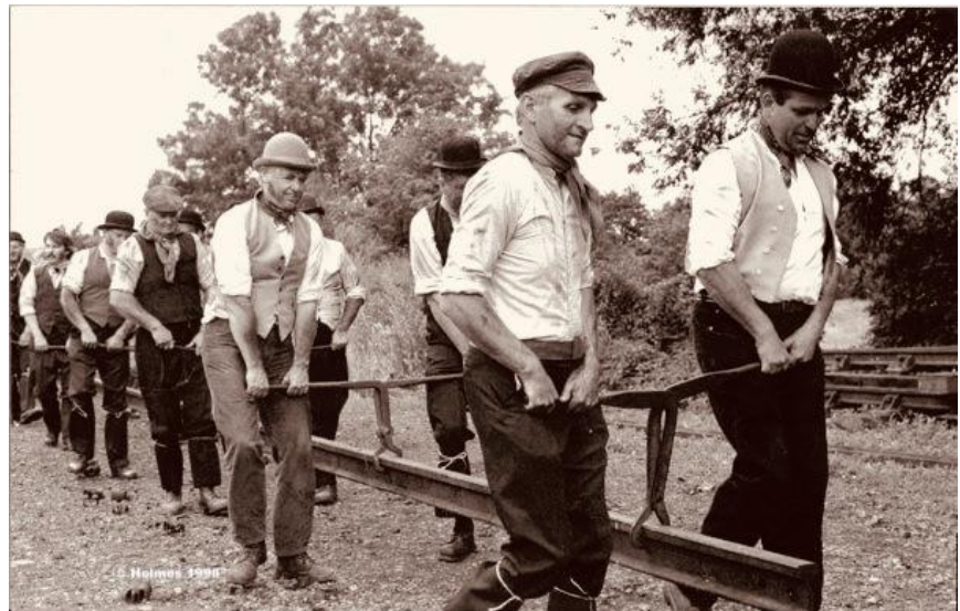
Close up of the nips fitting under the head of the rail.
