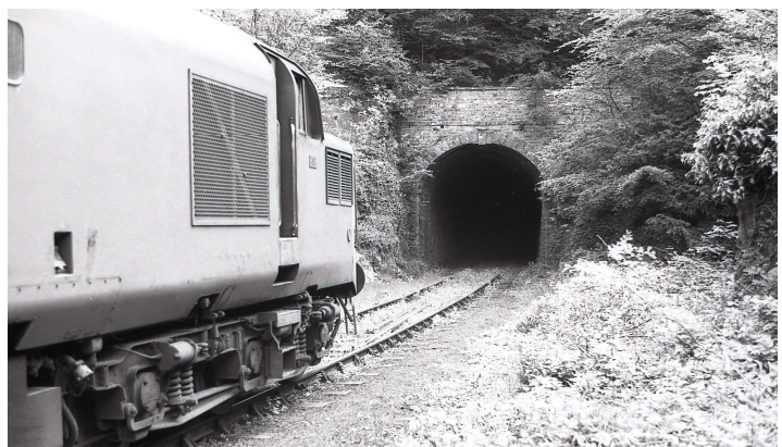
Northern portal Tidenham tunnel built by S W Yockney ( B.M. Handley)
